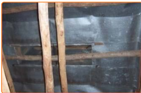
Barn Ceiling insulation with Paddy Straw
