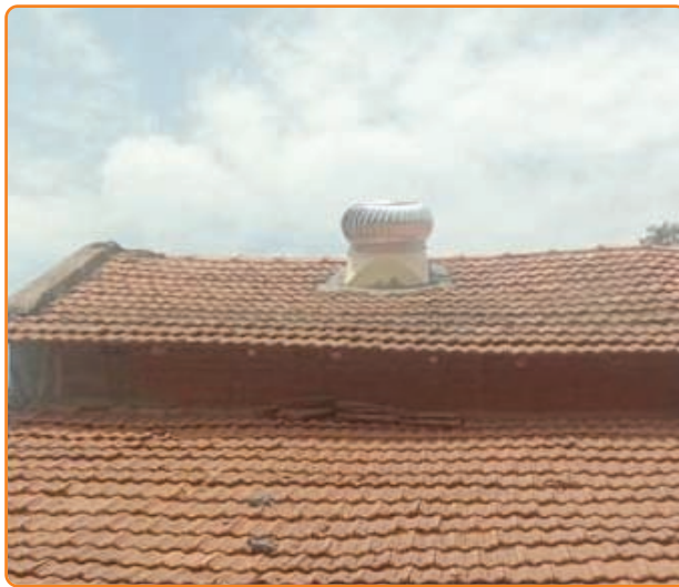
Turbo ventilator fitted Barn
